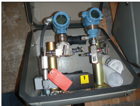
FIGURE 2. The use of transmitters with heating and isolation valving pre-assembled at the factory eases field installation
