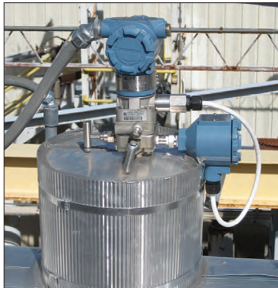
FIGURE 5A and 5B. In field installations with a transmitter on top, as shown in Figure 5A (left), the compact orifice integrated flowmeter is installed between existing flanges and eliminates heated sensing lines. In this installation, the use of wireless communication eliminates field wiring. For larger lines (Figure 5B, right), an averaging pitot tube is used to minimize pressure loss
