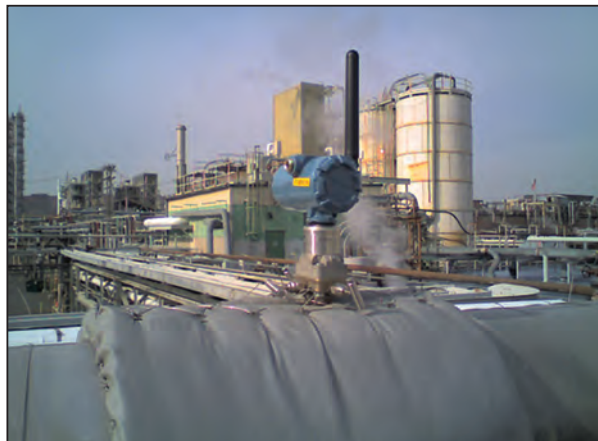
FIGURE 5A and 5B. In field installations with a transmitter on top, as shown in Figure 5A (left), the compact orifice integrated flowmeter is installed between existing flanges and eliminates heated sensing lines. In this installation, the use of wireless communication eliminates field wiring. For larger lines (Figure 5B, right), an averaging pitot tube is used to minimize pressure loss
